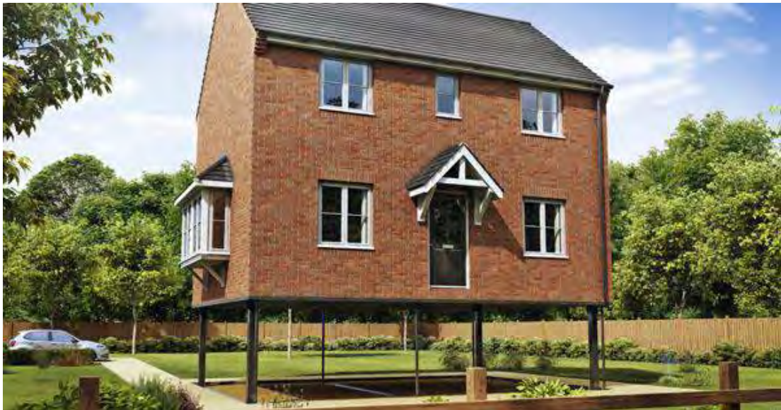
Figure 3: Larkfleet Home's elevating house.
